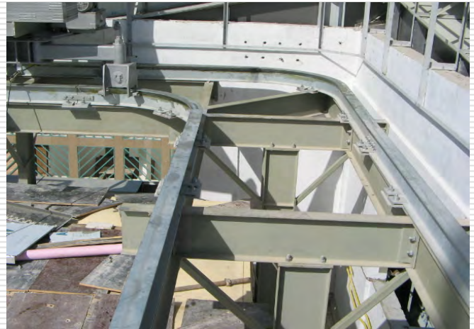
Tracks on Steel Structure
