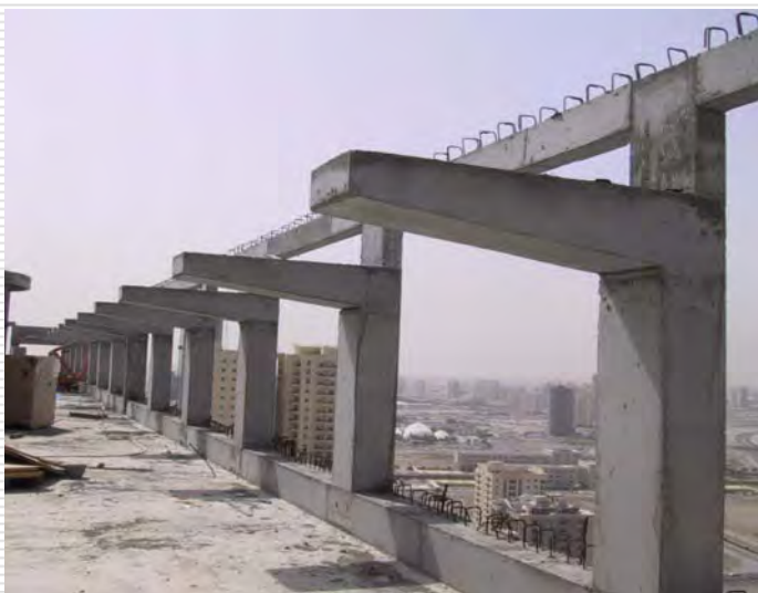
Elevated Up stands Structure
