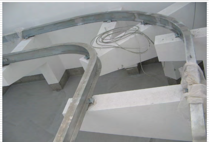
Tracks on Elevated Up stands
